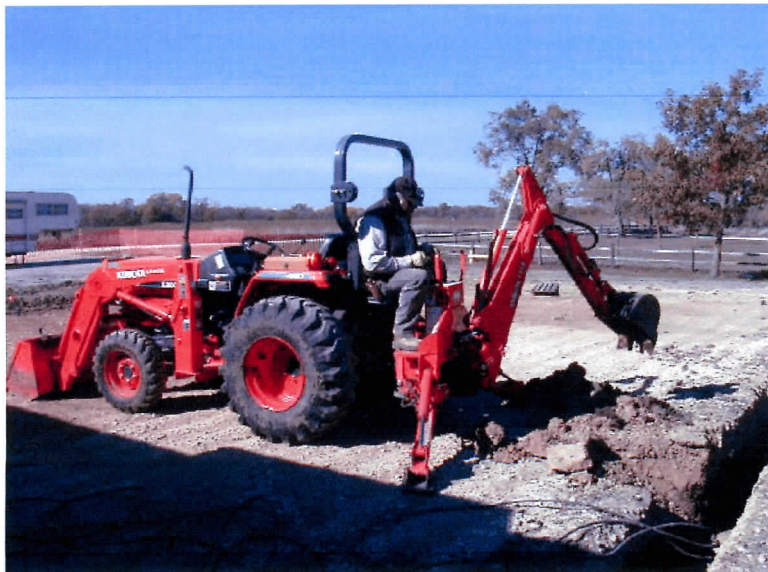
Gerald Laws using the baby backhoe, appropriately nicknamed "oh fuey", to clean out trenches at the expansion building site.
