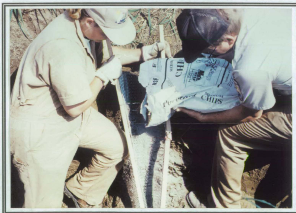
Figure 8. A wetland was restored on Kerbers WPA by filling an old well with bentonite.
