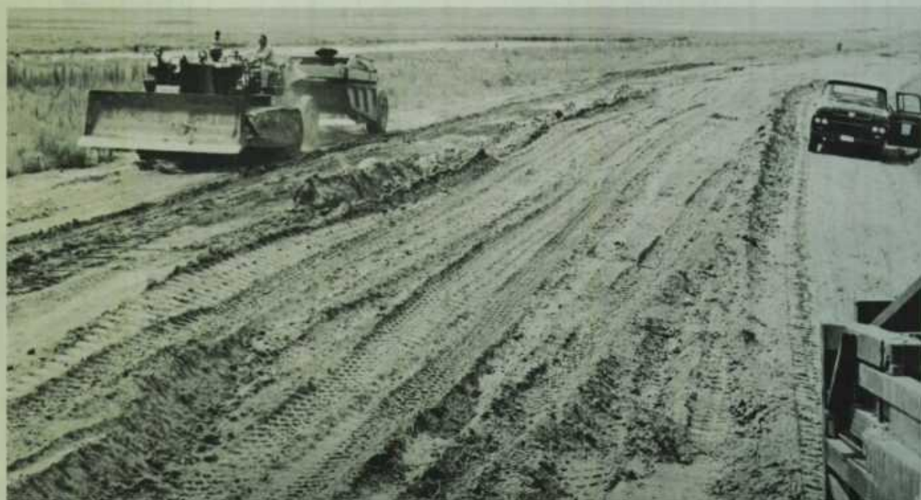
PROGRESSION. Construction of dikes along the reservoir shoreline forms rather large subimpoundments consisting of a network of sloughs in addition to other lands of various elevations above normal lake water levels.
