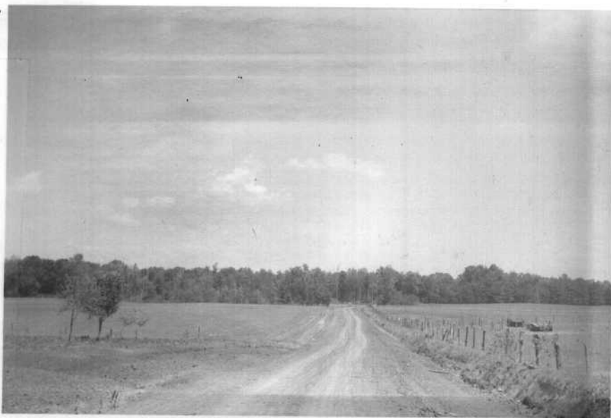
(1). White Springs Dike gravelling with stage of water in unit in background approximately 554.9 on gauge.
