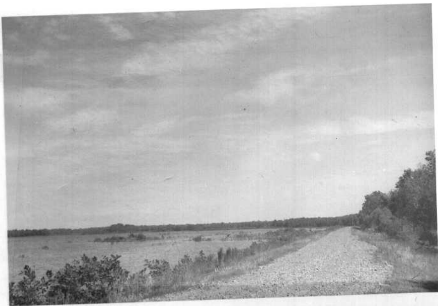
(1). White Springs Dike gravelling with stage of water in unit in background approximately 554.9 on gauge.
