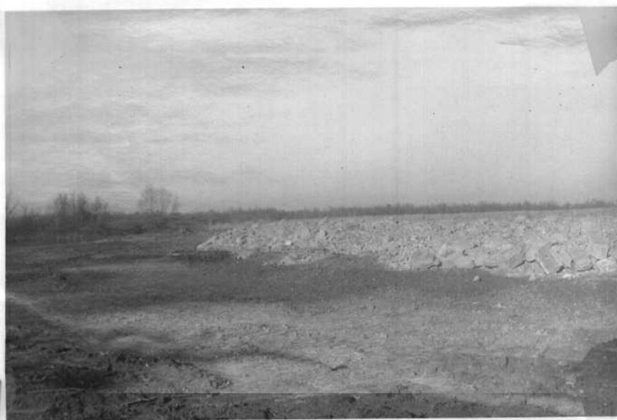
Photo No. 2. Section of White Springs dike - reservoir side-riprapped with crushed rock to correct or hold down erosion from wave action. Also, done in cooperation with T.V.A.
