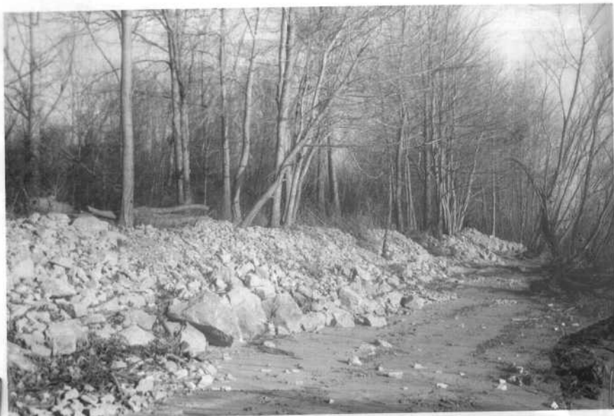
Photo No. 1. River bank protection - Adjacent east end of White Springs dike - in cooperation with T.V.A.
