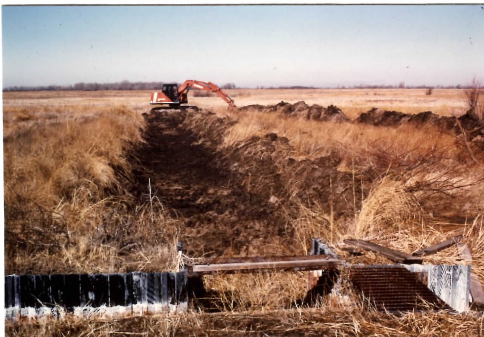
Figure 42. The borrowed Bantam excavator was used to construct a new ditch from the F-line canal into Unit 14B. 89-PG
