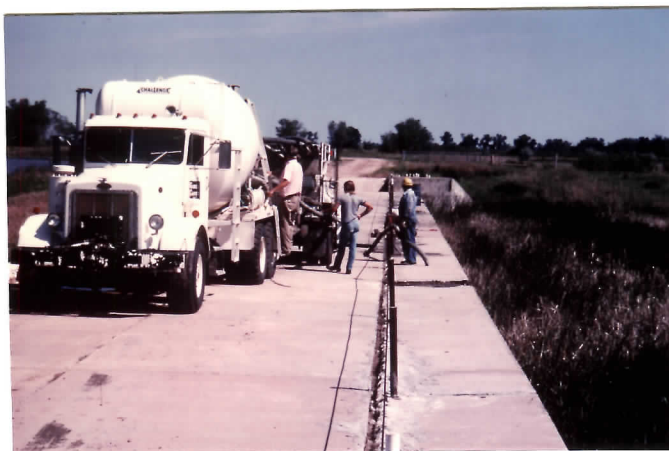
Figure 48. Concrete grout was pumped into the holes to fill the voids and strengthen the spillway.
