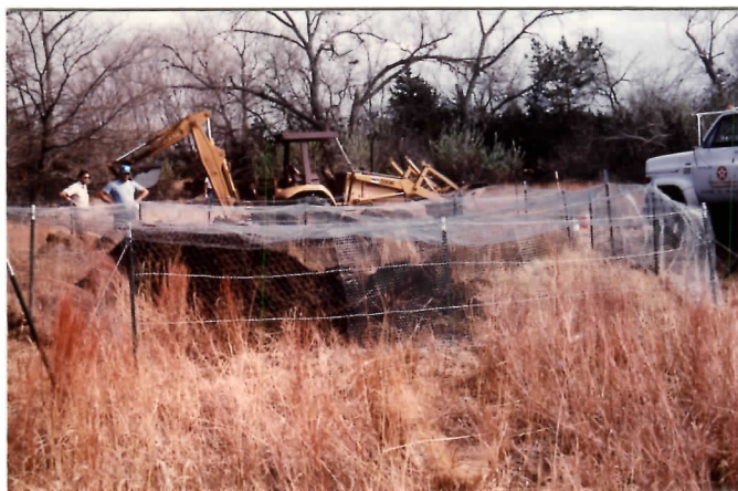
Figure 57. The area was fenced and a wire canopy installed to keep wildlife from entering the area. The seeping oil was pumped out and the contaminated soil was removed when the seepage had stopped. 89-DH
