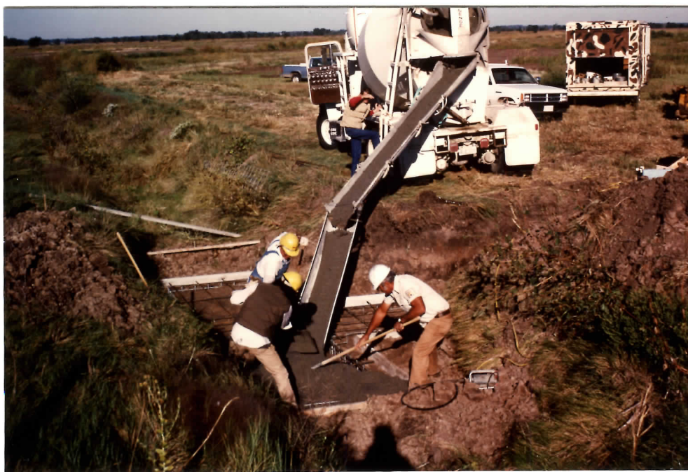
Figure 49. The new water control structure under development on Unit 30. Concrete structures with PVC pipes are far more durable in the refuge's corrosive soils than corrugated metal tubes. 89-PG
