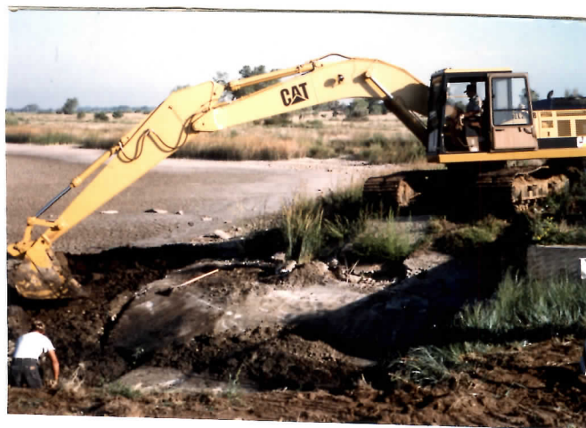
Figure 59. The new excavator was used to remove accumulated silt to start the structure repairs on the Little Salt Marsh. 91-BKM
