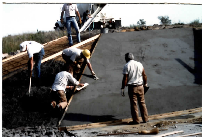
Figure 61. Pouring concrete on the steeply sloping walls was a challenge but the crew succeeded. 91-DRS
