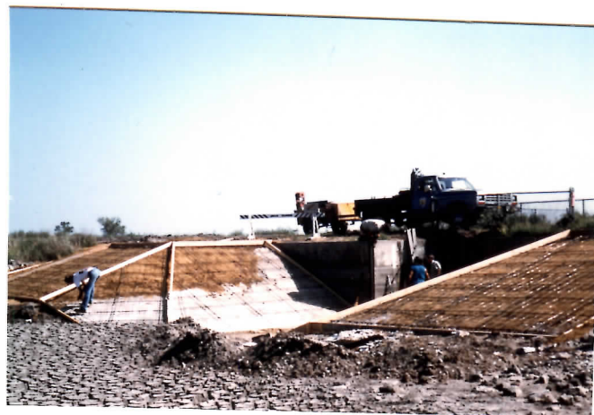
Figure 60. Concrete forms were installed to replace the deteriorated apron walls. 91-DRS
