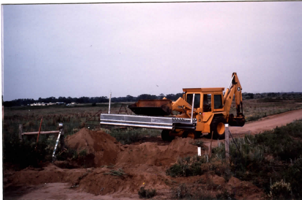
Figure 64. Using part of the $38,000 worth of surplus pipe we obtained in 1990, the crew built several cattleguards. The design does not require concrete supports and allows the guards to be somewhat portable. 91-DRS
