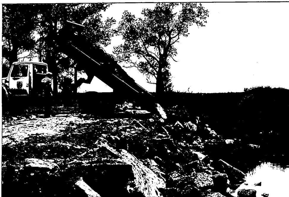
Figure 62. Part of the Reno County abandoned roadbed being used for rip-rap along Rattlesnake Creek to prevent erosion. 91-DH
