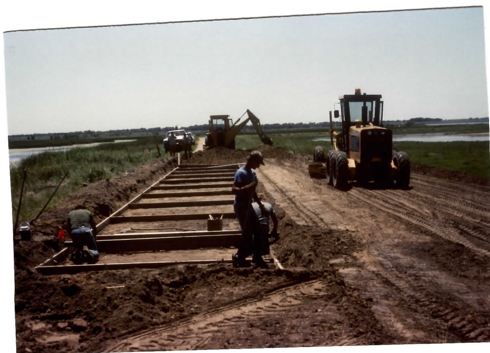
Figure 43. The refuge crew working on forming the new concrete spillway on Unit 58. New spoil was added and the spillways enlarged to provide better water movement. 92-DRS
