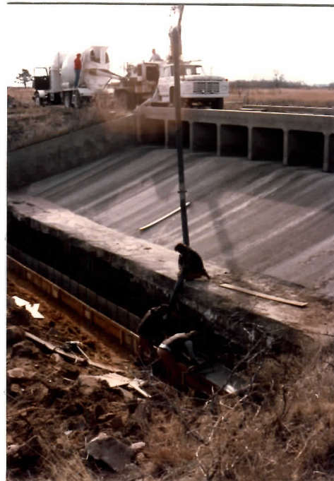
Figure 36. A new footing was poured for the Darrynane 9-Bay water control structure. 92-DRS
