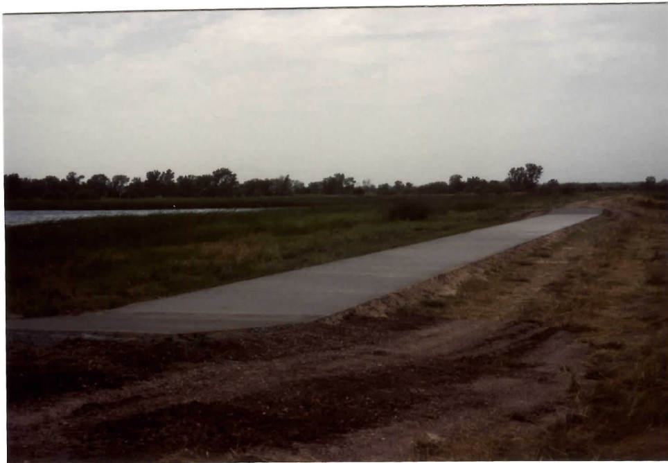
Figure 44. A new concrete spillway on Unit 11, replacing an earthen spillway and giving an extra margin of safety in a flood situation.
