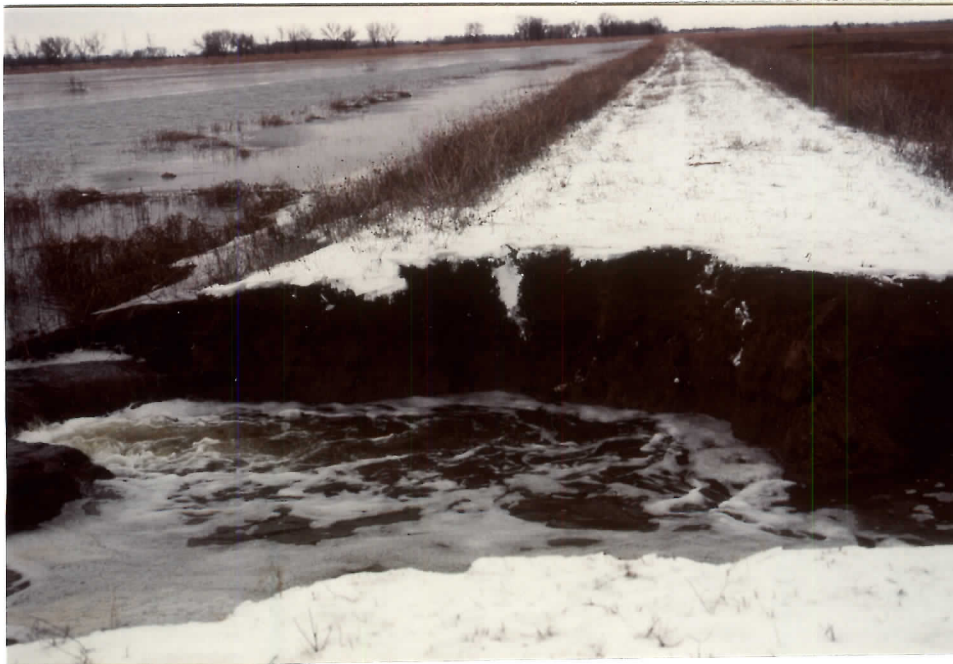
Figure 41. Part of the Marsh Road washout that resulted from the failure of the Unit 62 dike in December. 92-JDH
