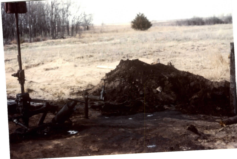
Figure 45. A lead line failed on Rama Oil Company's Quivira #10 well, resulting in a oil spill. The company cleaned up the spill and rehabed several facilities to prevent future occurrences.
