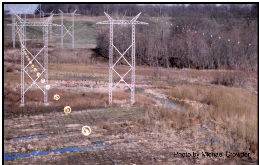
Photo 55 Swan Flight Diverters Installed at a 20-foot Interval in Indiana
