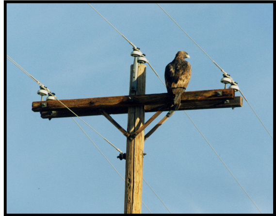
Photo 2 Golden Eagle and a Typical Three-Phase Tangent Structure
