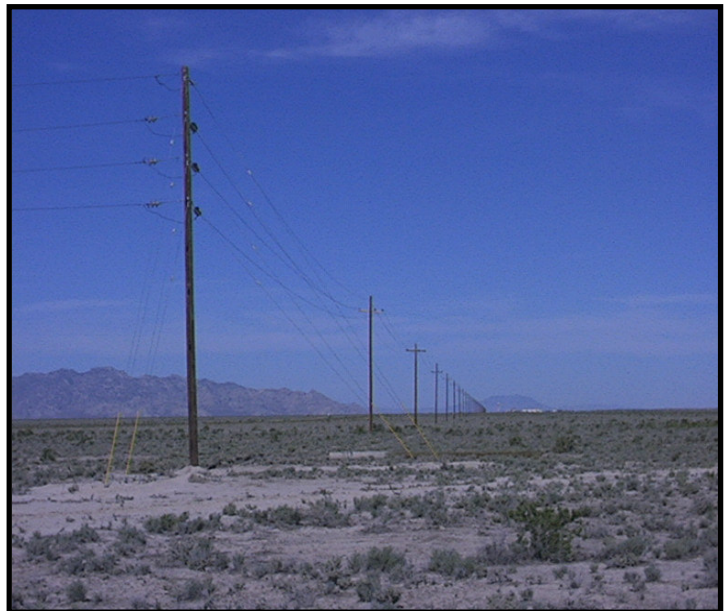
Photo 7 Three-Phase Vertical Bird-Friendly Angle Structure
