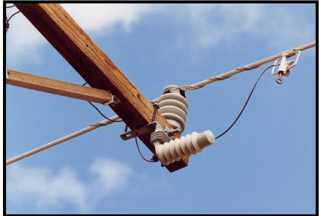
Photo 26 Horizontally Mounted Surge Arrester to Reduce Animal Exposure
