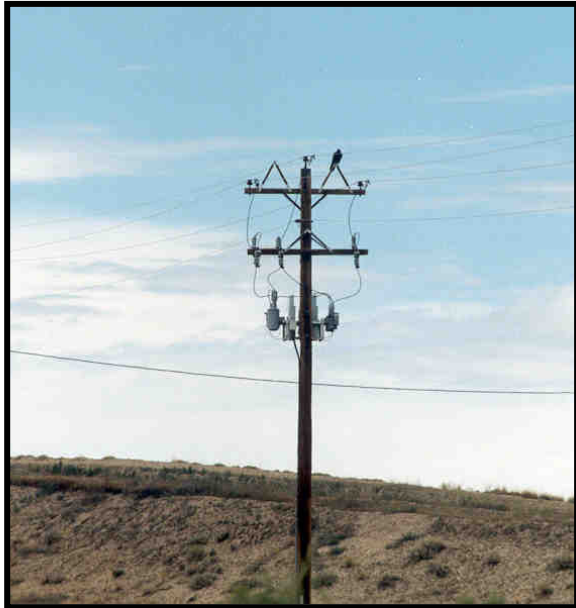
Photo 40 Bird Perching on a Triangle Perch Guard
