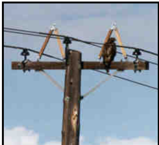
Photo 43 Raptor Perching under a Perch Guard
