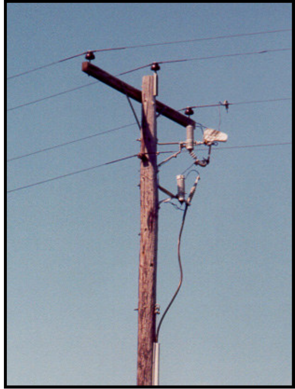
Photo 34 Single-Phase Metal Cutout/Arrester and Pothead Bracket
