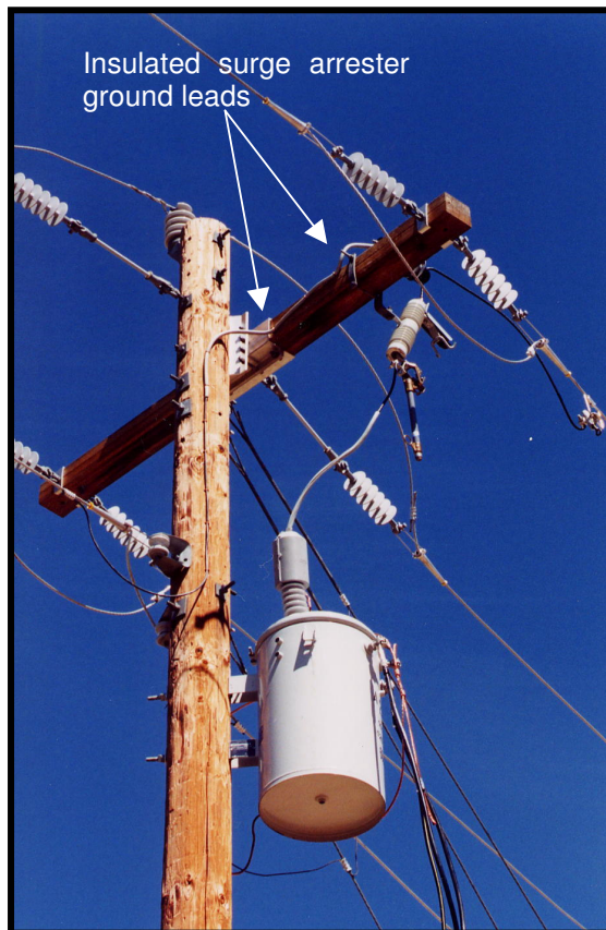
Photo 27 Insulated Surge Arrester Ground to Eliminate Phase-to-Ground Animal Contacts
