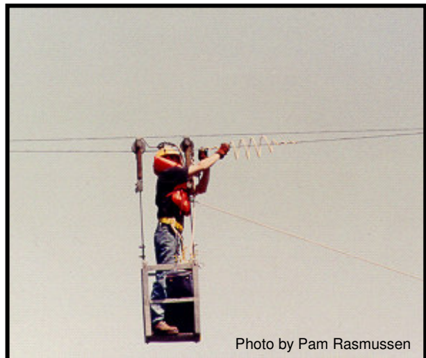
Photo 54 Lineman installing SFDs from a Suspended Pull Cart
