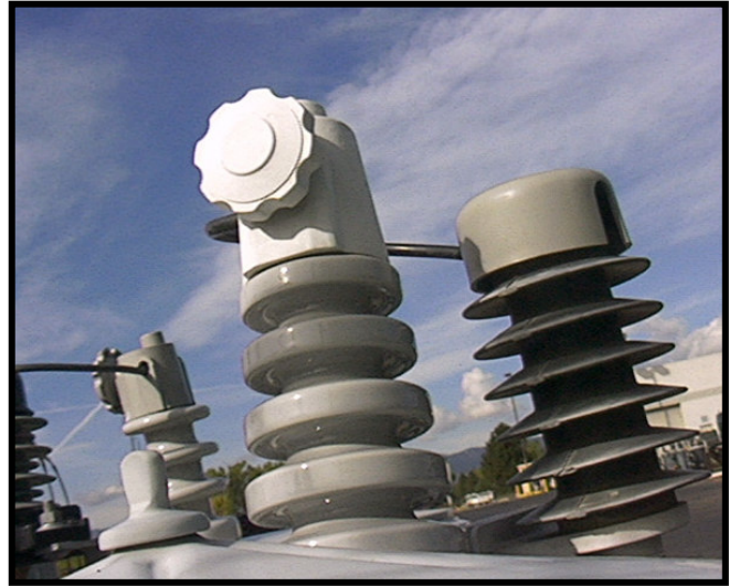
Photo 14 “Wheel-Type” Bushing Cover Delivered with the Transformer
