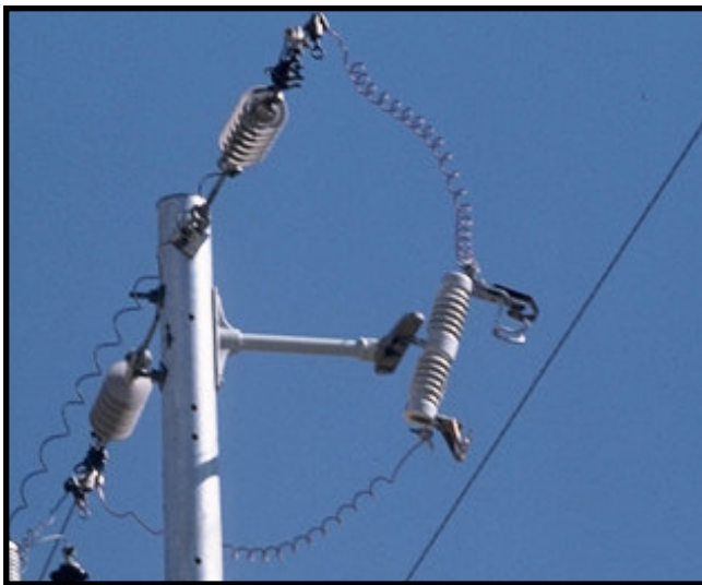
Photo 19 Cutout Mounted on an Insulated Fiberglass Bracket to Isolate Animal Contacts
