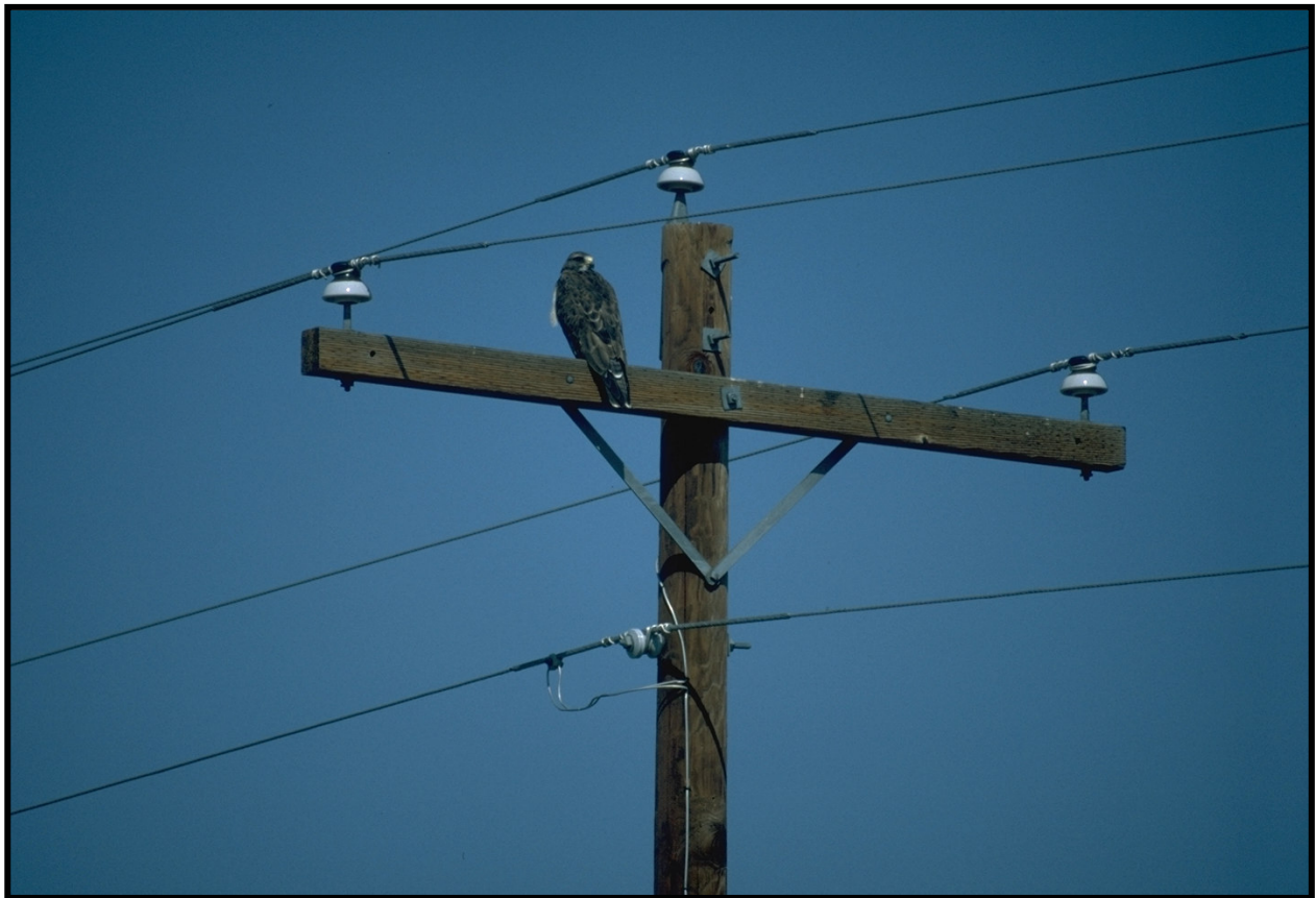
Photo 12 Swainson's Hawk Perching on a Crossarm Supported by an Ungrounded Metal Crossarm Brace
