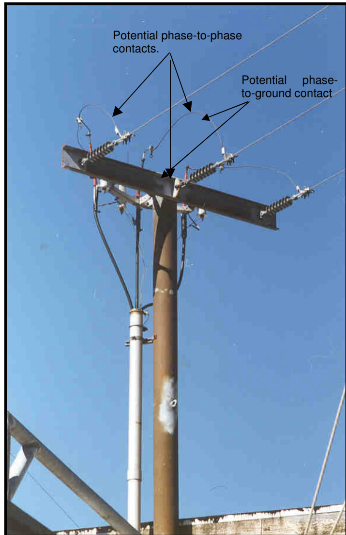
Photo 11 Metal Crossarm Posing a Significant Phase-to-Ground Electrocution Risk
