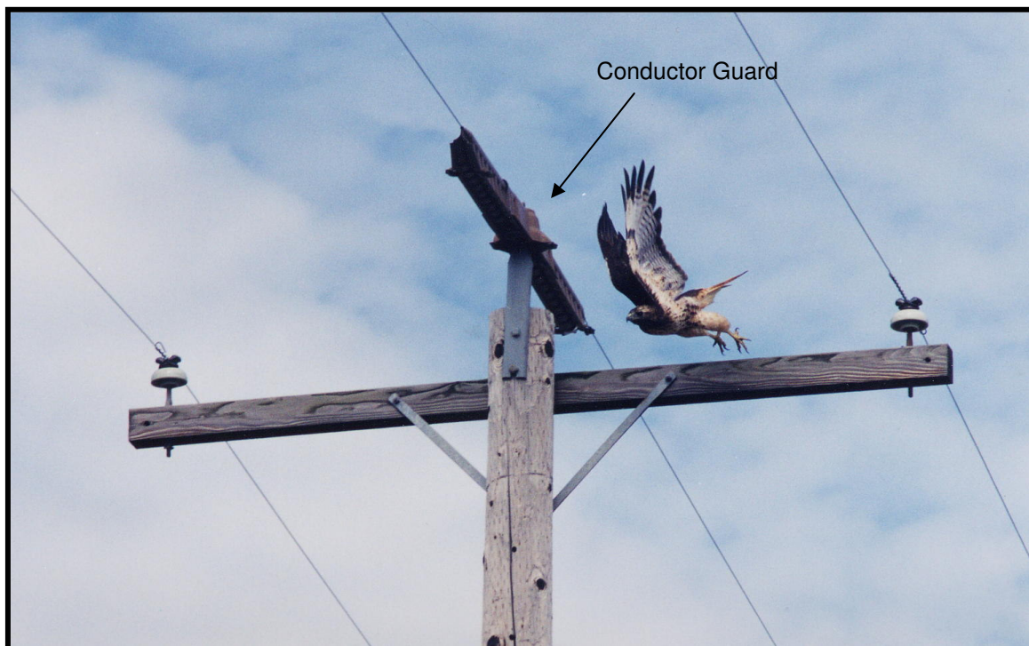
Photo 3 Kaddas Bird Guard Mounted on a Preferred Perch Structure
