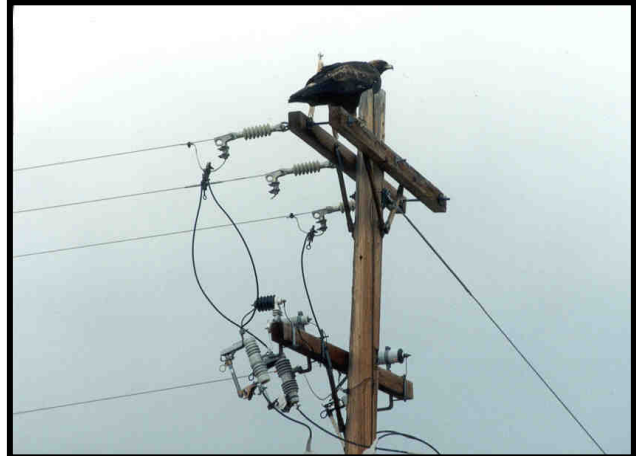
Photo 41 Perch Guard Shifting an Eagle Toward the Safe Side of a Deadend Unit
