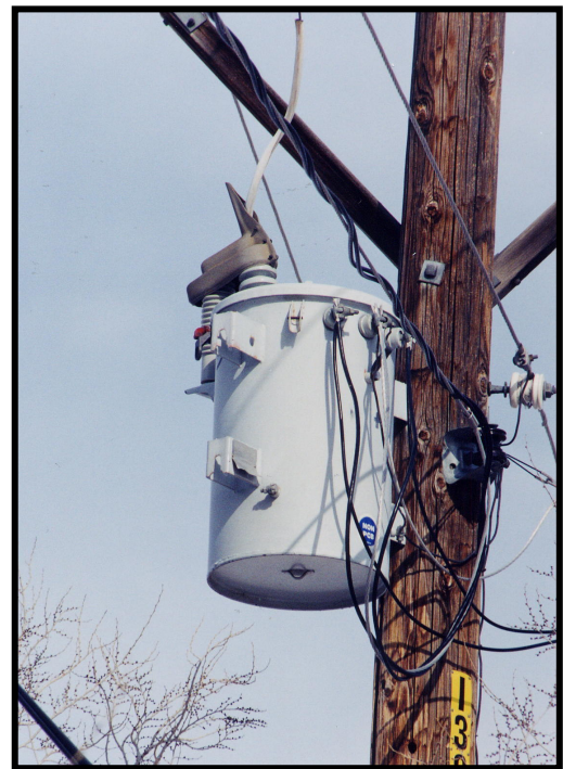
Photo 17 Combination Arrester/ Bushing Cover
