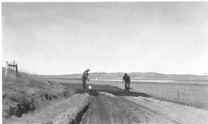
Spreading loam on road
