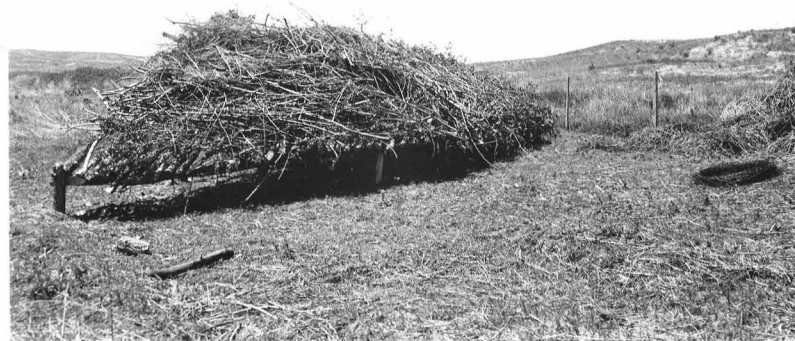
NE-CRL-113 These shelters are being rebuilt, bringing the back to the ground, leaving only small escape openings
