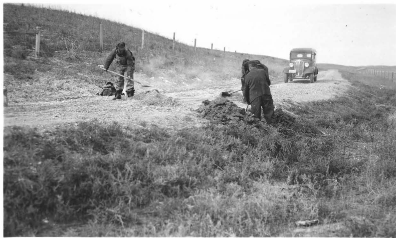
The start of a culvert to drain road
