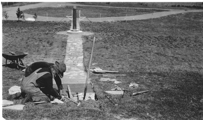
NE-CRL-095 Flag pole base complete, with walk
