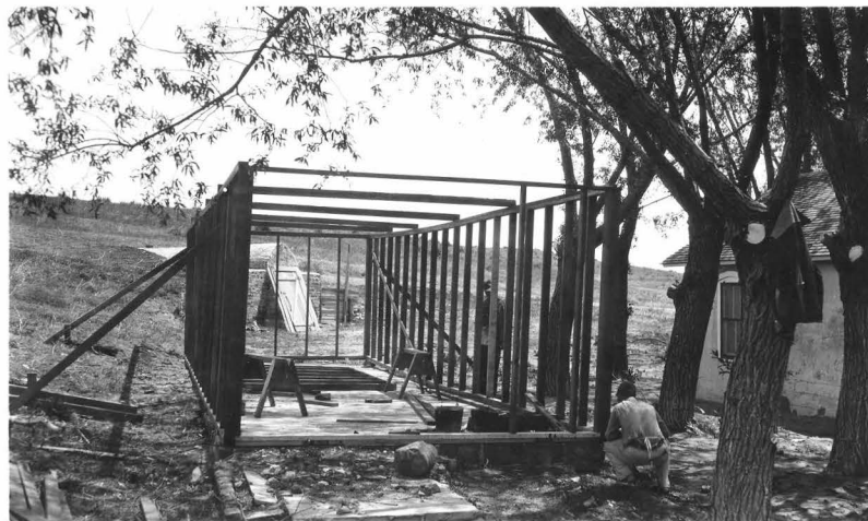
Building of garage and fuel shed on the above platform
