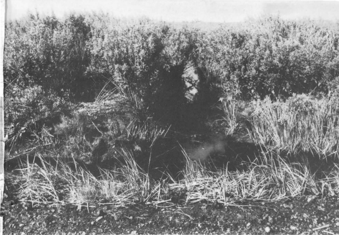
Figure 20.—View of South Bowers marsh, Kent County, Del., showing the results of an attempt to control mosquito breeding by "sump" drainage. From the "sump" a ditch was dug to an outlet to Murderkill River, but was plugged with the board structure seen in the foreground. Muskrats cut around this structure and "sump" drainage became "gravity" drainage. This resulted in the destruction of the marsh, including three ponds of appreciable size and some smaller ones containing luxuriant growths of wigeongrass, and accommodating quite a few waterfowl during the migratory season. The marsh proper has been taken over by impenetrable thickets of Baccharis and Iva . August 1946.
