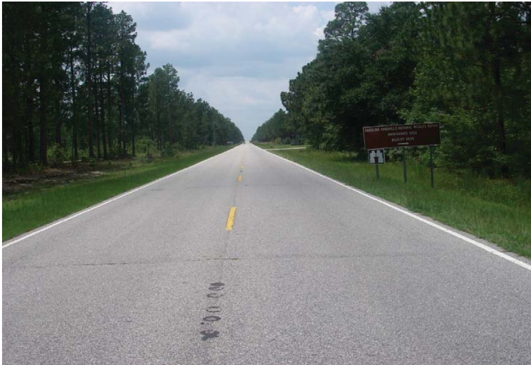
Photo 2: The Carolina Sandhills National Wildlife Refuge Maintenance Area Wildlife Drive sign does not conform to the MUTCD, and also sign restricts sight distance looking northbound.
