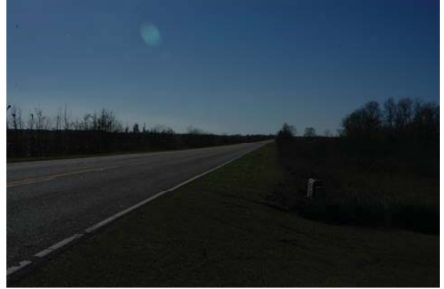
View of SC-170 near the entrance to the Savannah NWR maintenance facility. Photo shows the lack of shoulders and guardrail as well as the drop-off from the roadway into the wetlands.
