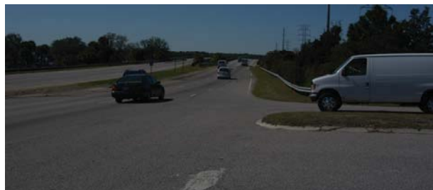
View of US-278 westbound from the entrance to the Pinckney Island NWR. Photo shows the limited acceleration lane for vehicles entering US-278.
