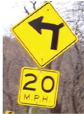
Photo shows an example warning sign that could be used to warn motorists of the entrance to the Laurel Hill Wildlife Drive. The speed advisory plaque should be based on current roadway conditions. There is currently a 45mph curve advisory sign near the entrance to Laurel Hill.
