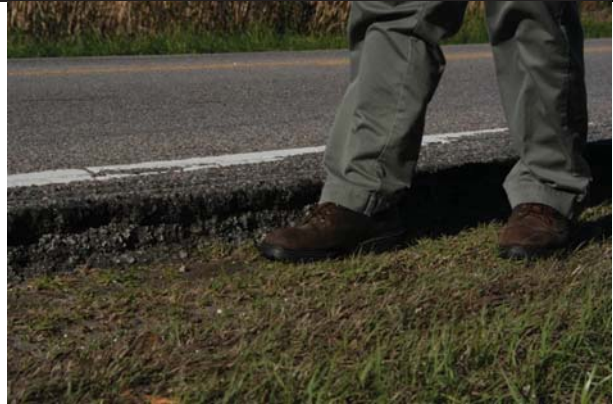
Example of large pavement edge drop-off along SC-170 near the entrance to the Laurel Hill Wildlife Drive.
