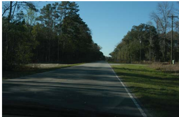
View of US-17 near the new visitor center. The photo shows the entrance to the new visitor center on the left and Sawgrass St. on the right. The photo illustrates that there appears to be space (not necessarily right-of-way) to provide turn lanes for the entrance and the residential street.
