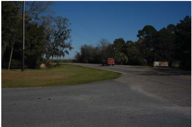
View of the entrance to the Savannah NWR maintenance facility. Photo shows that the entrance is located near a horizontal curve, which limits the view of the entrance from SC-170.
