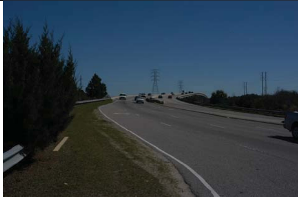
View of US-278 to the east of the entrance to Pinckney Island NWR. Photo shows the horizontal and vertical curvature that limit sight distance near the entrance.
