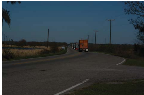
View of SC-170 eastbound. Photo shows the lack of paved and unpaved shoulders, particularly along the horizontal curve. The photo also illustrates the significant truck traffic along this route.
