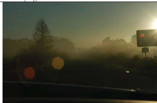
Photo shows the effect of fog and glare along SC-170 in the early morning hours. Roadway alignment is difficult to see as are roadway signs.
