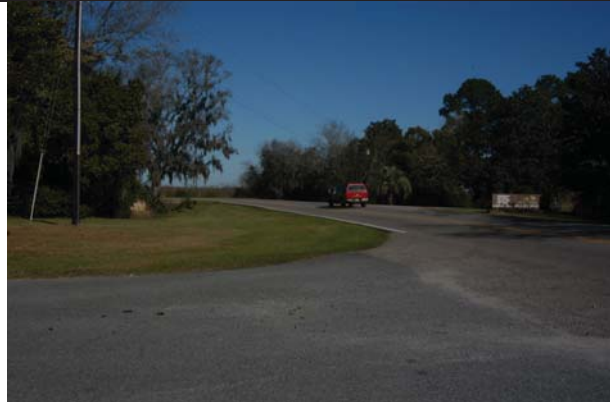
View of access points to maintenance facility and Savannah NWR wildlife drive. This photo illustrates the lack of turn lanes at the access points and the horizontal curve that limits sight distance.
