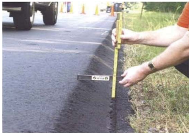
Photo shows an example of a safety edge. The beveled edge is installed at a 30 degree angle.
