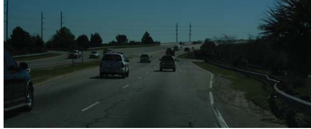
View of US-278 eastbound just prior to the entrance of Pinckney Island. There is a right- and left-turn lane from US-278, but the lengths are relatively short. The photo also shows one of the nearby bridges that restricts the length of turn lanes in the westbound direction.
