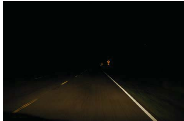
Photo shows a relatively good example of a section with retroreflective pavement markings and high-intensity signs.
