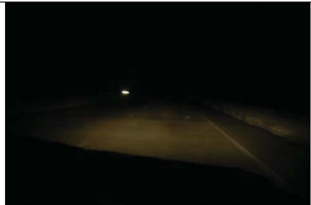
View along study section of US-278 at night. Photo shows the lack of nighttime guidance due to the faded pavement markings and lack of raised pavement markers along the centerline.
