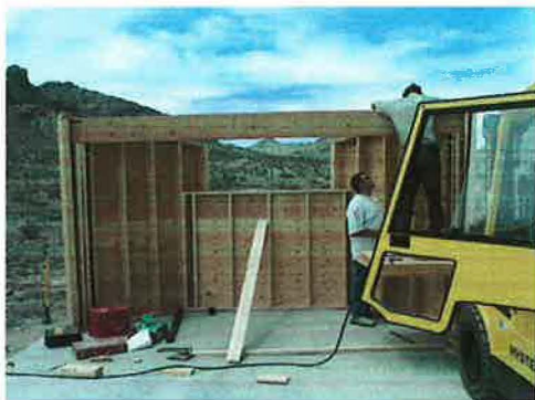
Fig.21 Construction of new kiosk at main refuge entrance.
