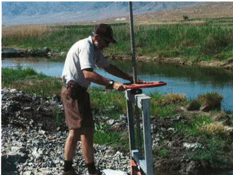
Fig.9. Unidentified field person opening newly constructed screw gate at structure #8.
