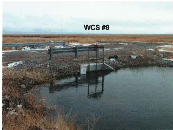
Fig.28. Newly constructed water control structures with screw gates attached.
