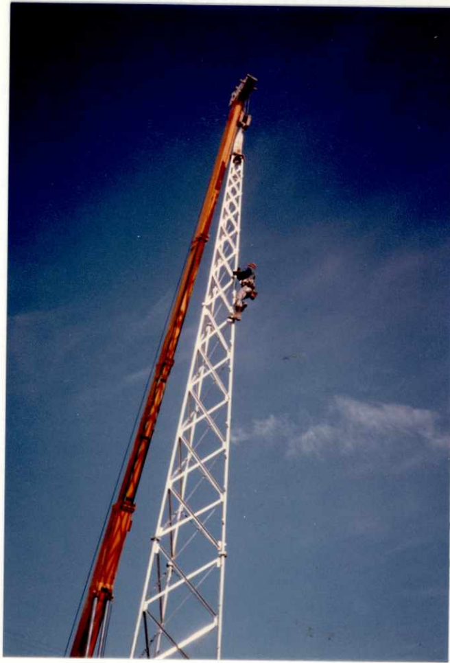
A 4 kw wind generator was installed in early 1982. Here the tower is being erected.
