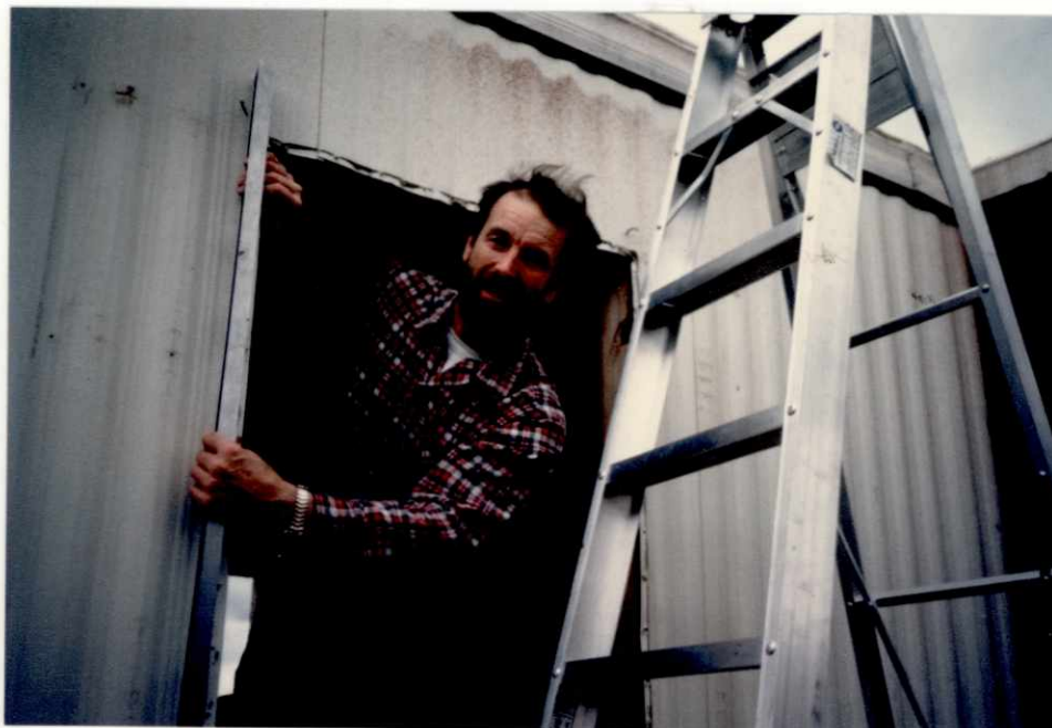
Glen Miller provided expert maintenance and soothing music during his tenure from June - September. Here Glen is preparing to replace uninsulated windows in one of the refuge trailers with thermopane windows, a welcomed addition.
