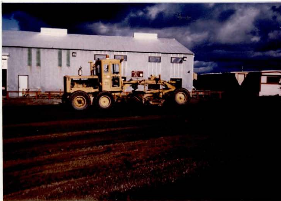
U.S. Air Force grading new gravel in the Refuge Office parking area.
