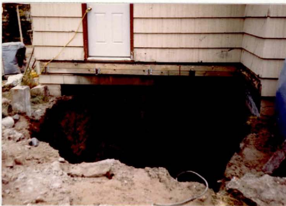
Excavation site after the leaking fuel tank was removed.
