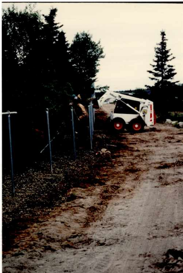
RO Construction Team of Walt, Harold and Bill in the process of installing the new chain-link fence on the west compound boundary.
