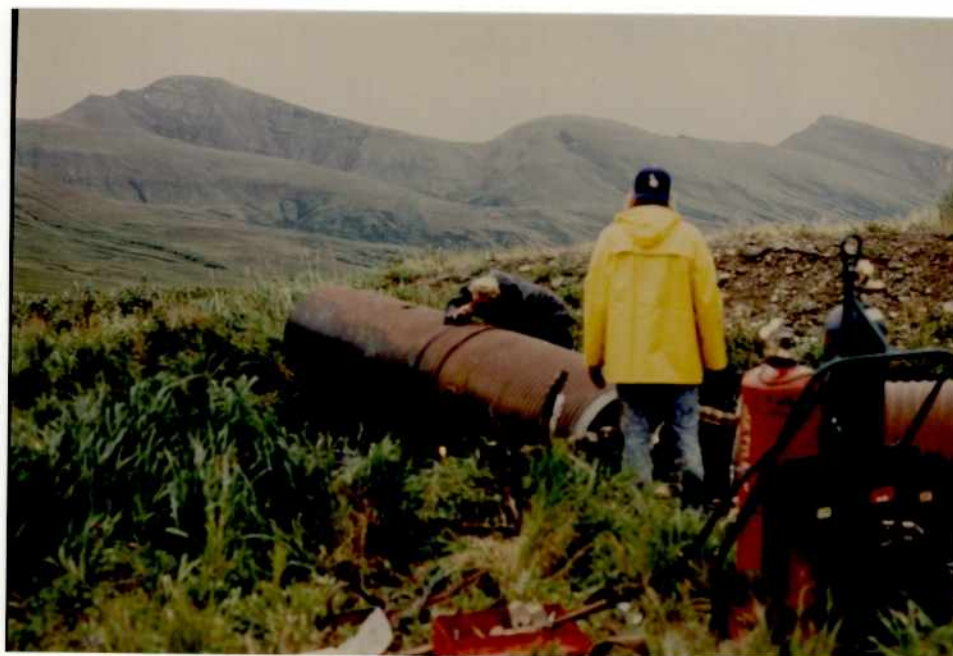
Exxon cleanup crew working on a culvert section preparing it for removal by helicopter.
