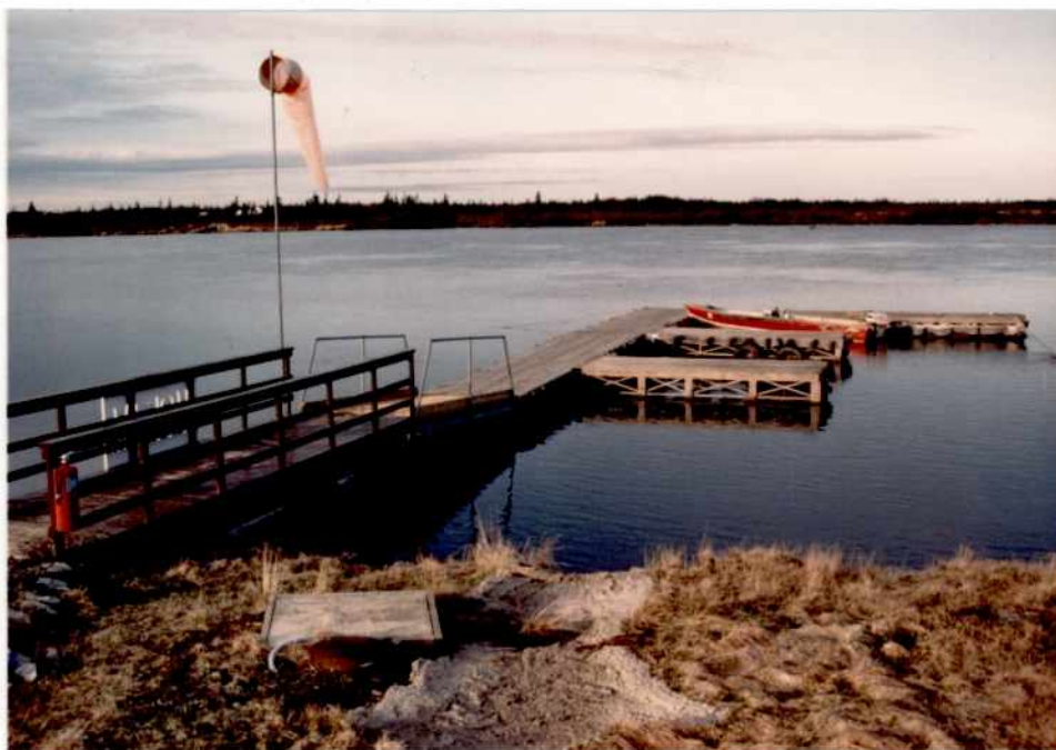
This view shows the entire dock, utilizing the new assembly system. Note the lack of poles no longer needed to drive into the riverbed to hold the dock in place.
