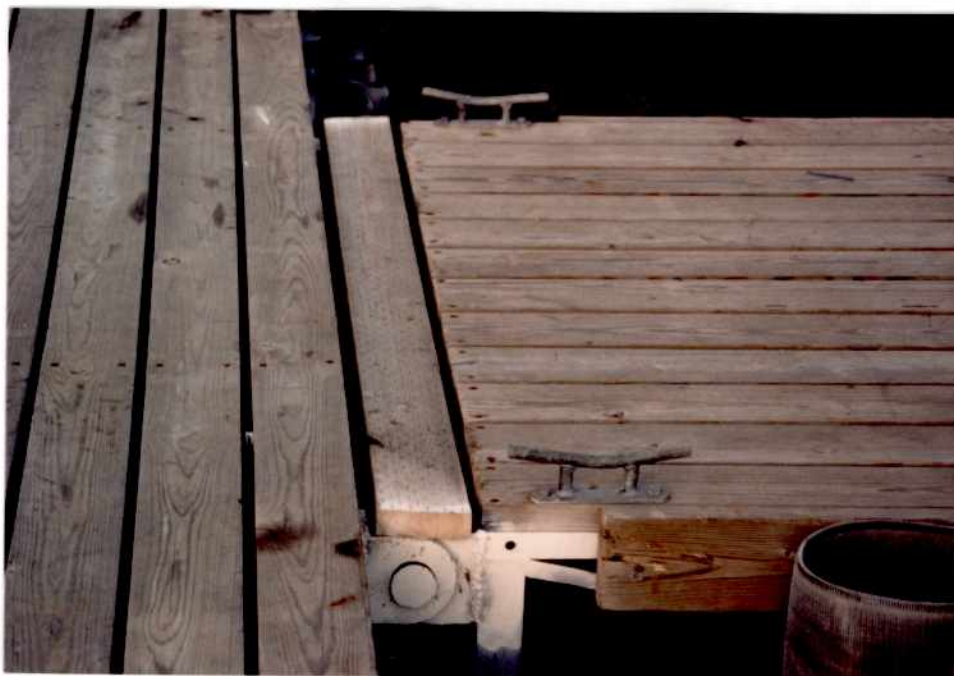
This new "pinning system", invented by MW Terry significantly improved the ease of putting the dock in and out of the river.
