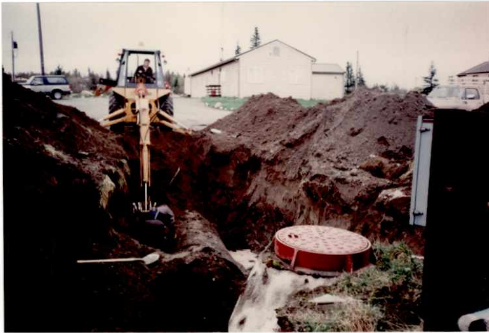
Maintenance staff removing old septic system at Headquarters. 05/94, RDP
