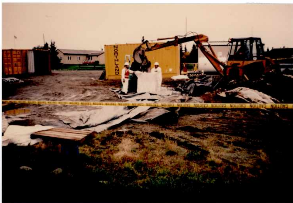
Contractor's in action, bagging fuel "contaminated" soil for shipment by barge in the yellow container vans to Lower 48.
