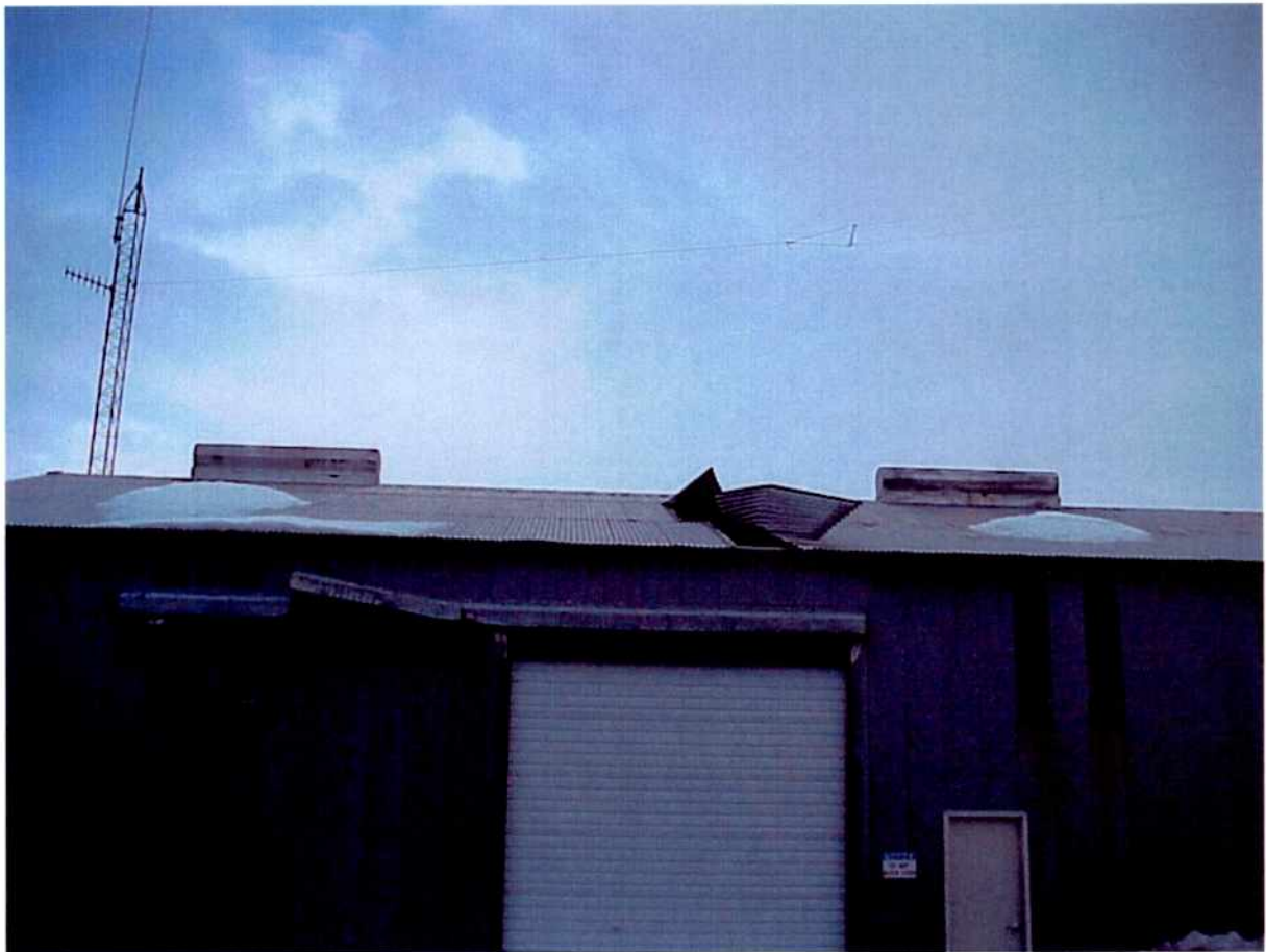
Wind damage to building 4.
