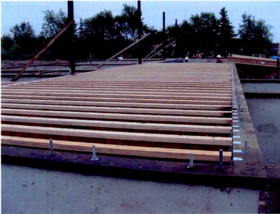
The first floor floor joists are added.
