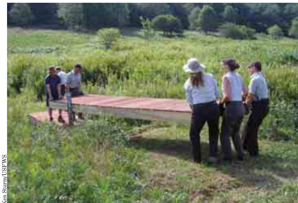
Installing a bridge over Glade Run
