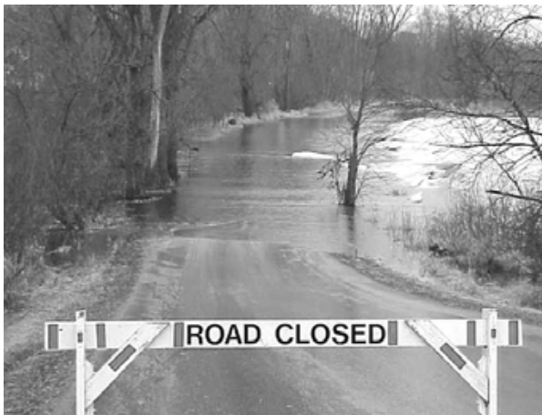
The main access road into Trempealeau NWR floods annually. USFWS
