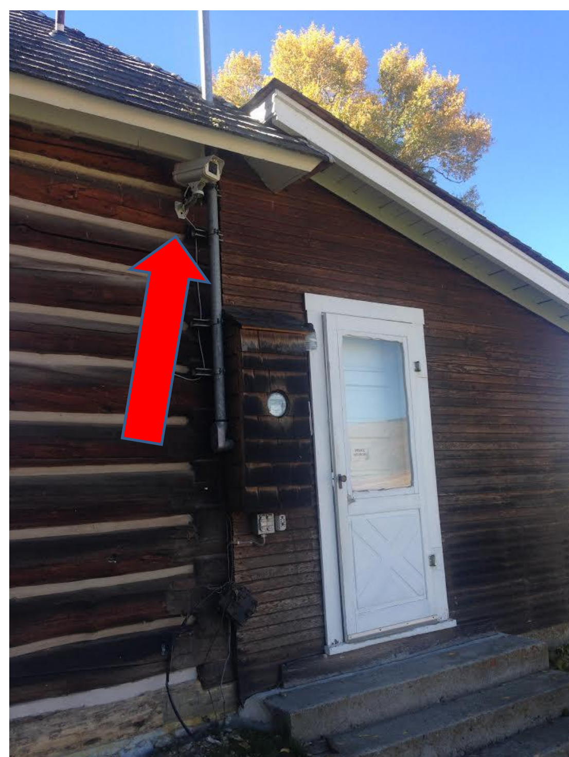
Figure 1 National Elk Refuge PhenoCam camera on historic Miller House. Installation includes IR enabled security camera with automatic web upload capabilities.
