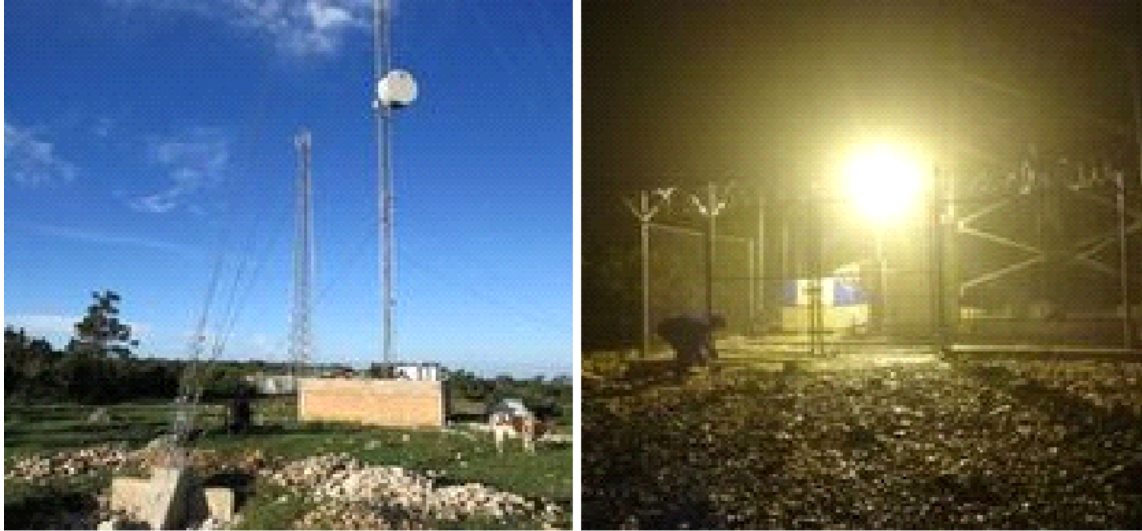
Figure 2.12. Communication towers near Black-capped petrel nesting areas on Hispaniola. Height of structures and associated guy wires depicted in left image; nighttime security lights depicted in right image. A disoriented and grounded Black-capped petrel also being recovered from the ground in right image. Photos by J. Goetz.
