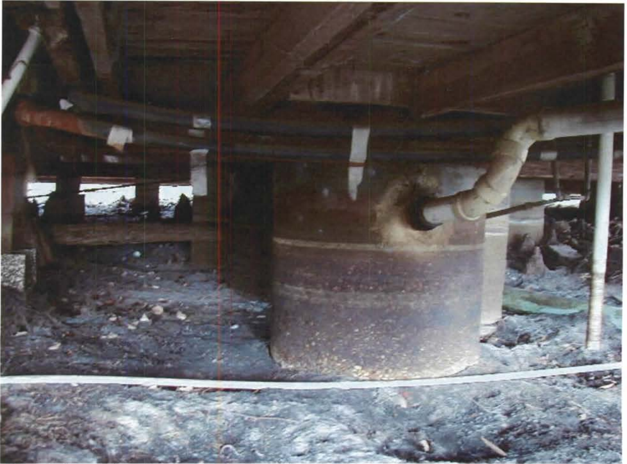
Figure 1. Exposed septic system at Banks Lake.
