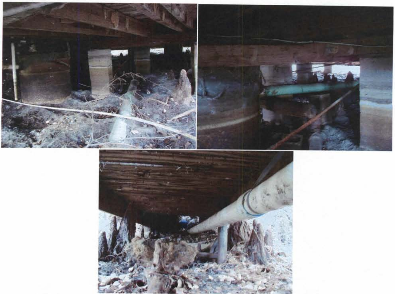
Figure 3. Exposed septic systems at Banks Lake.
