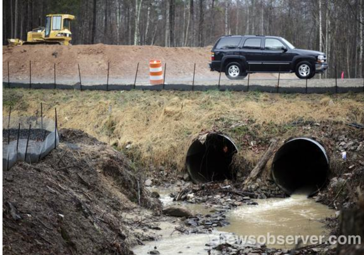
Figure 4-6 Perched culvert (credit: Raleigh News and Observer)
