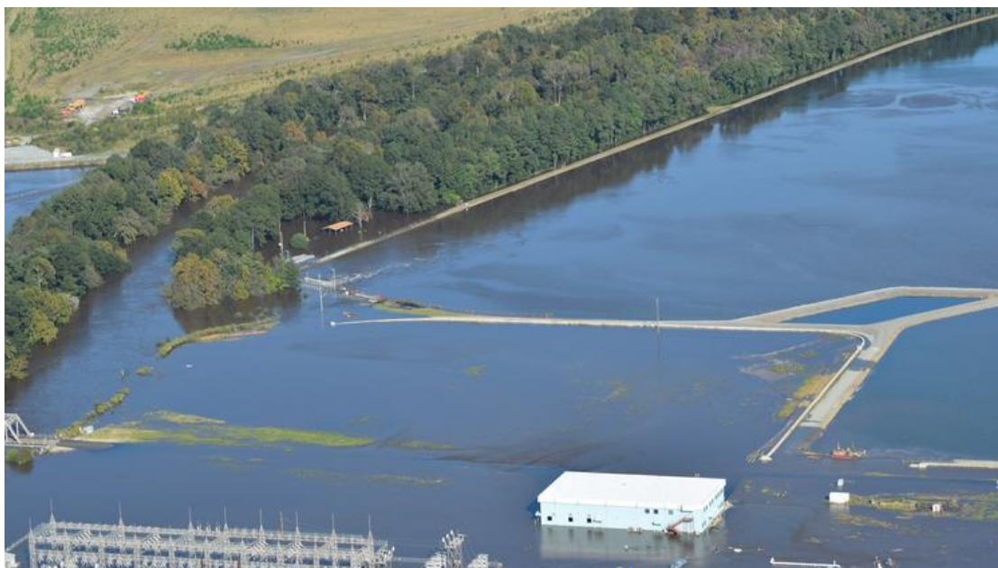
Figure 4-10 Hurricane Matthew: rising waters from Neuse River inundate coal ash storage pond near Goldsboro, NC (credit: Travis Graves, lower Neuse Riverkeeper)
