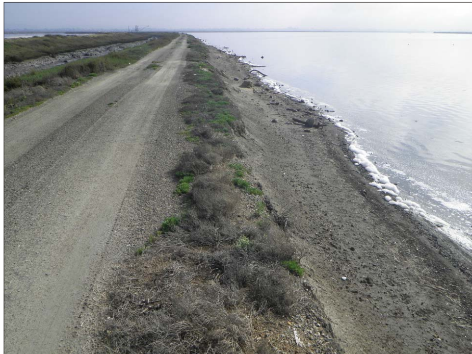
Photo 1: View of typical salt pond levee conditions (March 13, 2013)
