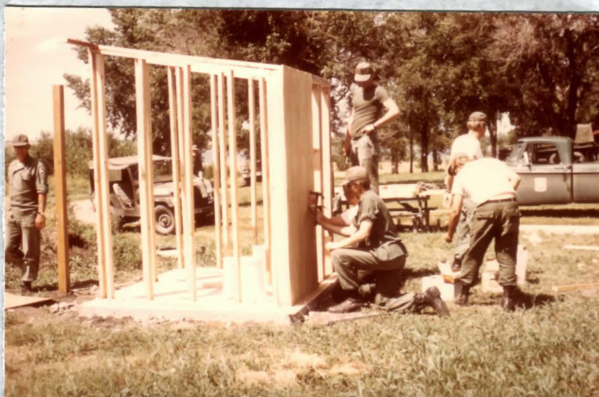
National Guard 153rd Engineer Battalion constructing vault toilet. Stone 8/14/72, 72-8
