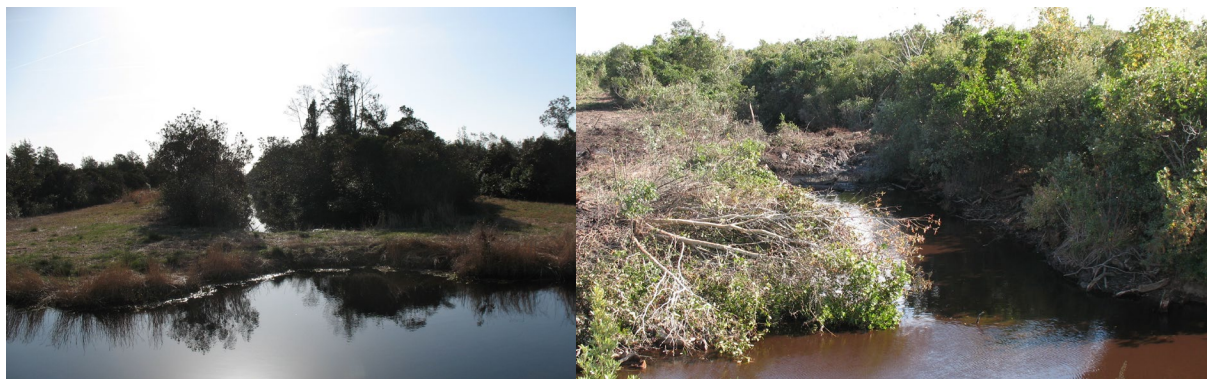
Figure A-13. Earthen plugs used to block water flow in a ditch/canal.
