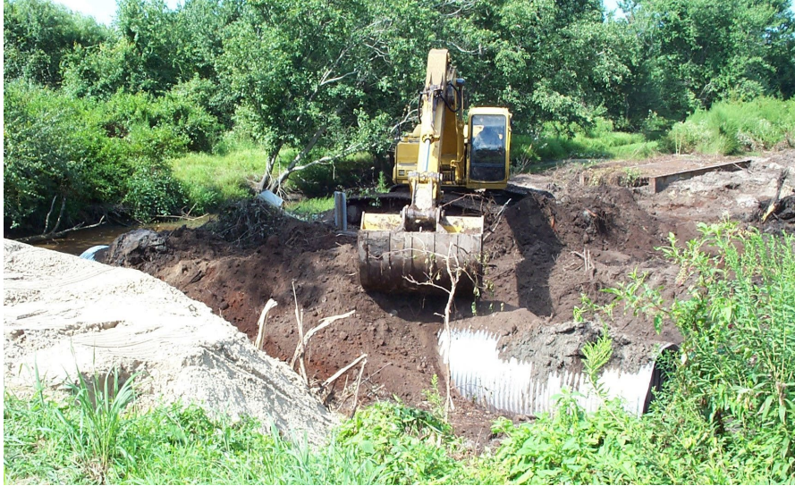
Figure A-14. Culvert installation.
