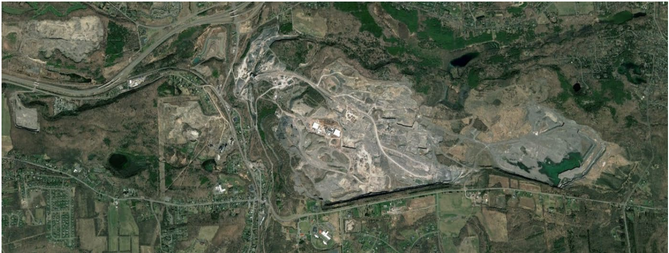
Figure 4-2. Aerial image of the Onondaga Escarpment in New York. The large quarry in the middle of the image removed three populations of the AHTF, and the majority of all AHTF populations in New York occur either to the east or west of this quarry.
