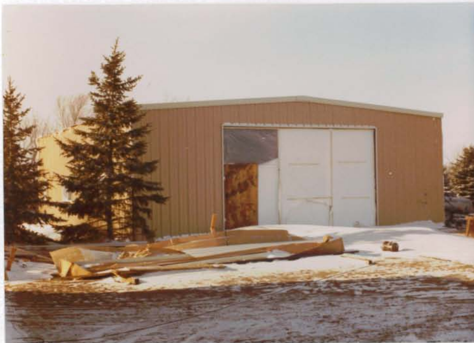
Fine, new shop nearing completion.
