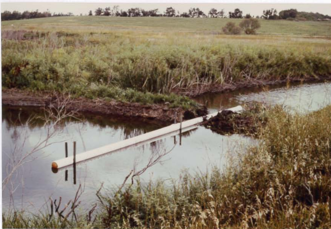
Refuge personnel installed this tube through a beaver dam to lower the water level and eliminate flooding on a neighbor's farm field. DJB - 7/87
