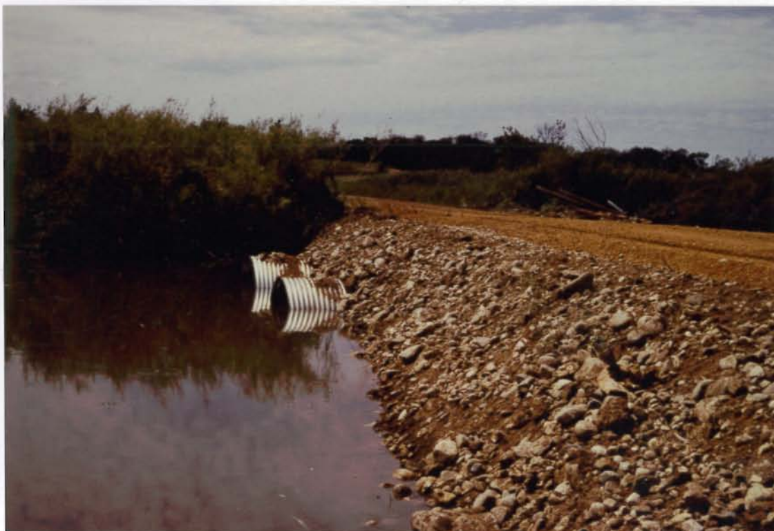
Sargent County replaced an unsafe bridge with these two new culverts in 1987. DJB - 7/87
