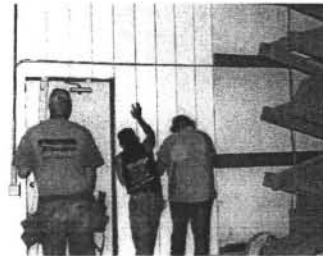
Contractors installing panel liners
