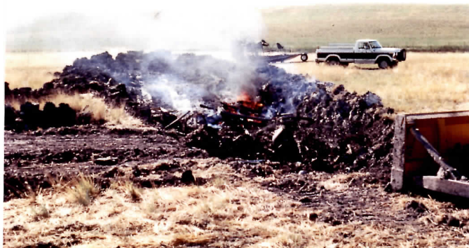
Fence removal in the lake was facilitated by the airboat. Posts and wire were burned and buried.
