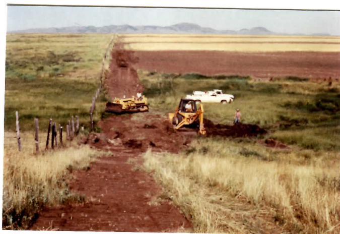
During Road construction began with installation of a 48 inch culvert. 81-19-14 WB
