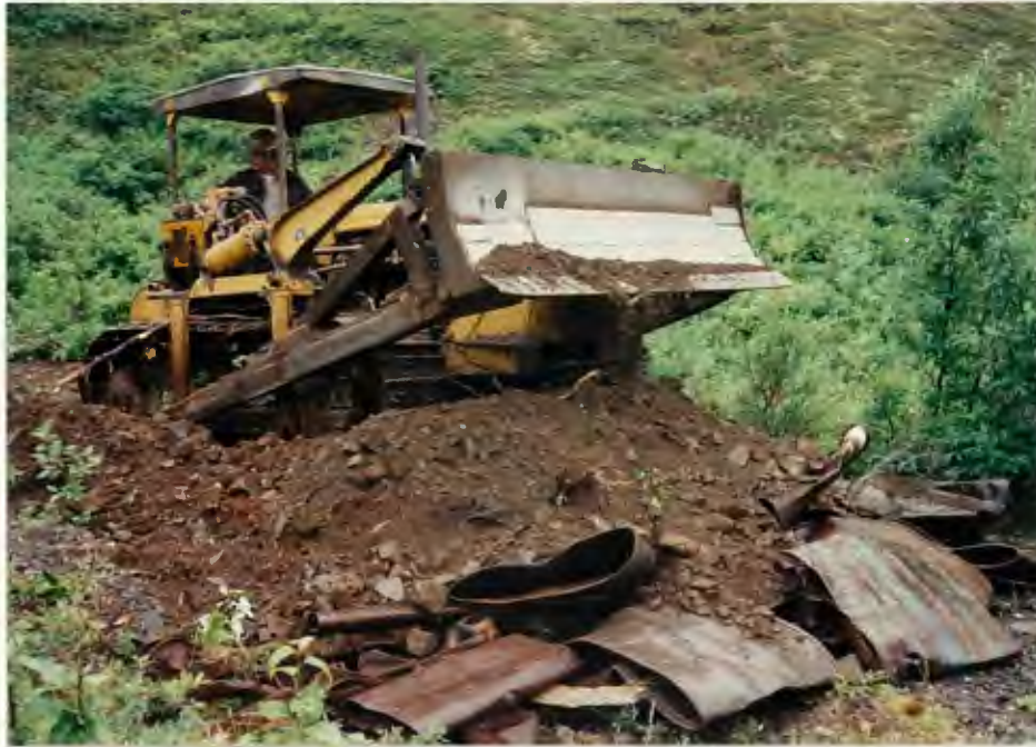
Bulldozer being used to flatten and then bury drums at the Canyon Creek mine cleanup site. (Rick Hubbell)
