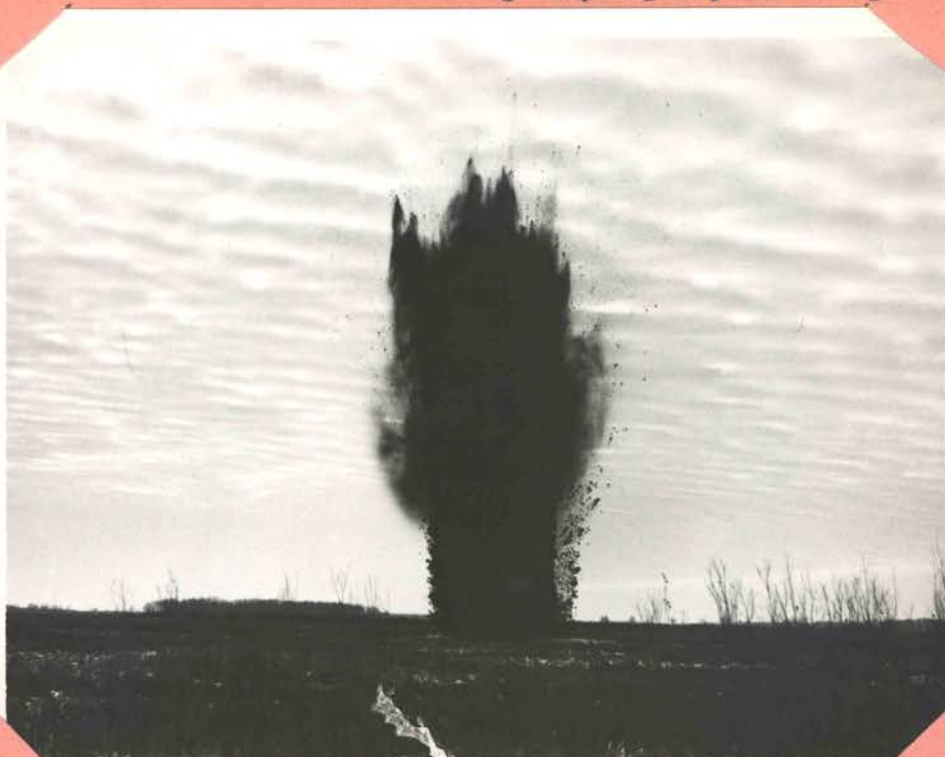
Monsanto Blasting Agent was easy to handle and showed good results. Eight holes were blown in sedge-cattail flats.
