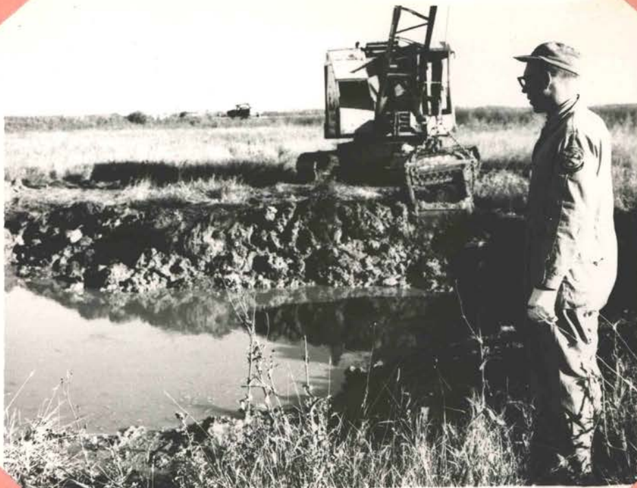
Erickson checks progress of pothole construction on west gate development site; 30 were dragline dug with 200' spacing.
