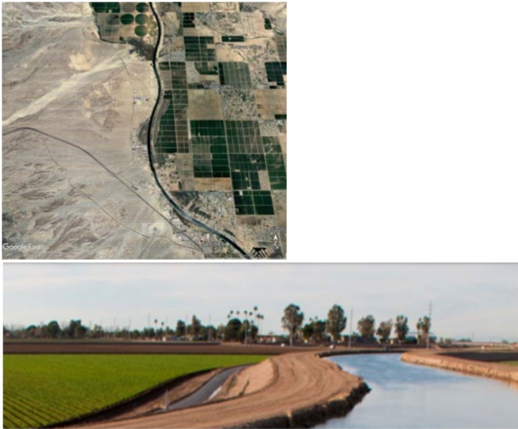
Figure 19. Lower Colorado River mainstem channelization, levee, and river bank armoring. Top photo is south of Davis Dam at Needle, AZ. Lower photo is near the international border with Mexico near Yuma, AZ (image from U.S. Bureau of Reclamation Yuma Division website).
