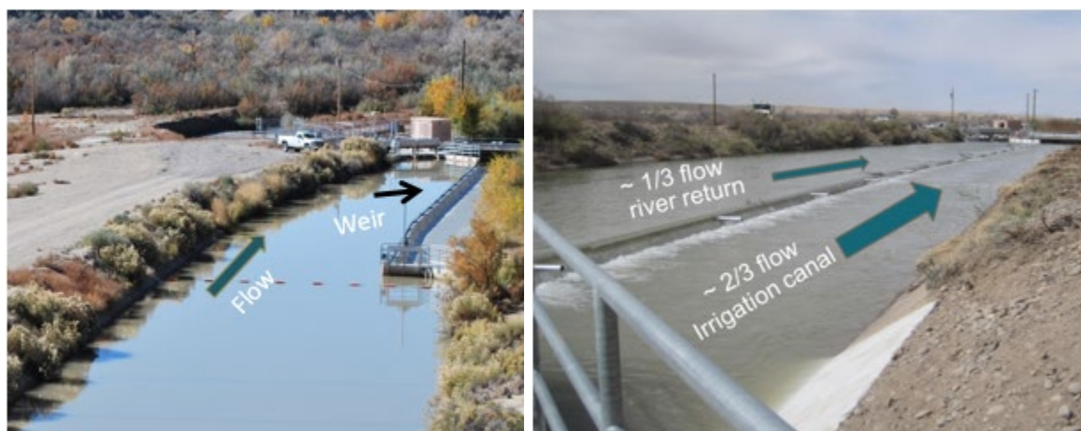
Figure 35. Weir wall installed in 2013 to reduce fish entrainment into the Hogback irrigation canal of the San Juan River (images from Brandenburg et al. 2017).
