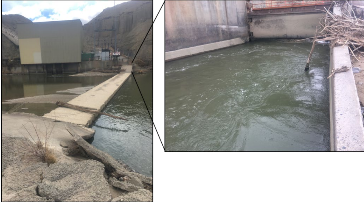
Figure 34. Arizona Public Service weir (left) and sluiceway (right) on the San Juan River, March 2018. Photos courtesy M. McKinstry.
