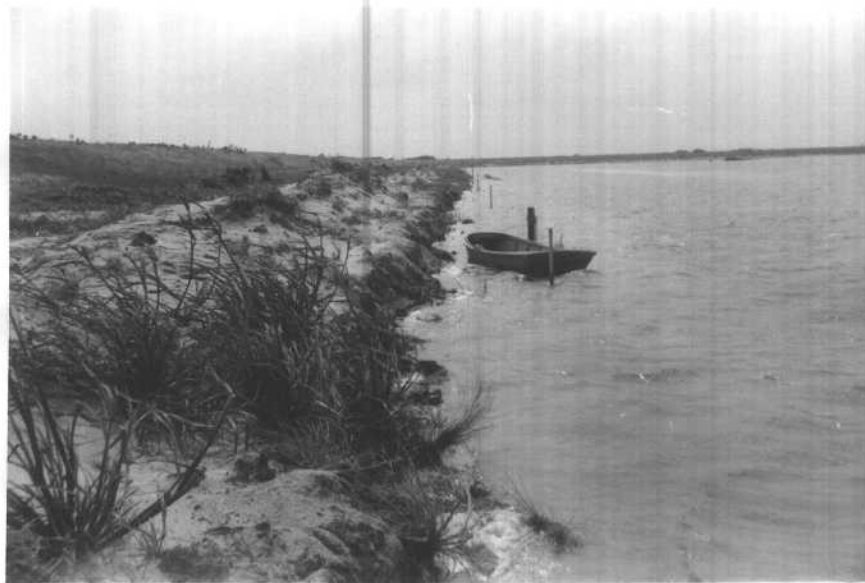
2. Same location as above, Summer of 1960 after dragline rebuilding.
