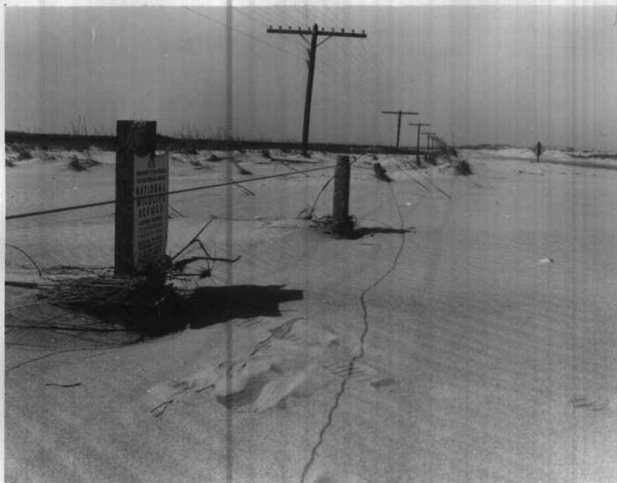
Sand was deposited along the fence line and in some cases completely over the fence posts.
