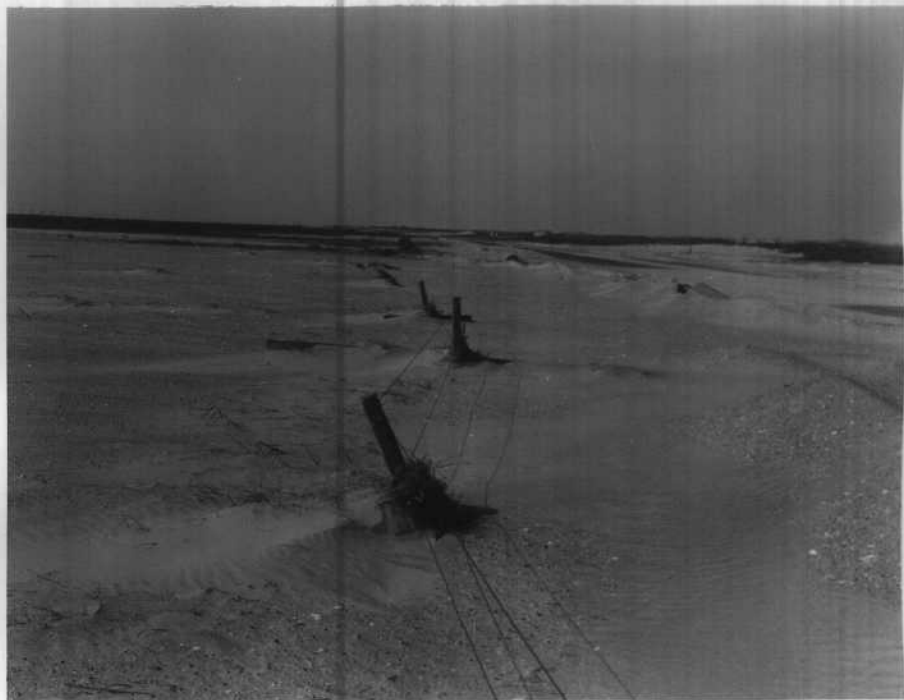
The fence line was badly damaged where the sand and water crossed from the east side of the public road to the west or marsh side of the road.
