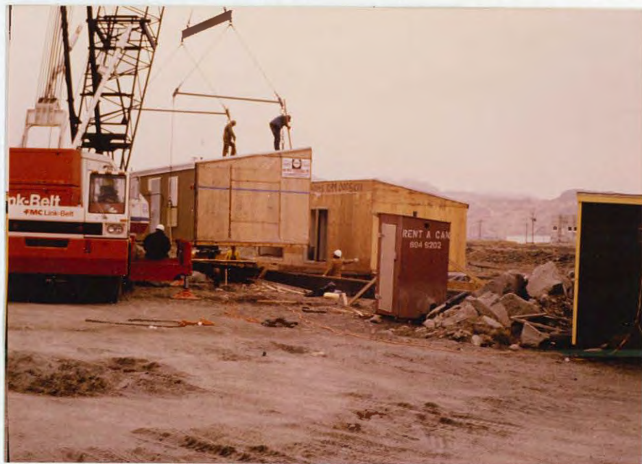
A duplex "half" being lowered into place. (J.M. 1981)
