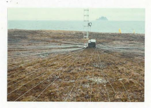
Ground view of a typical Navigational tower site on St. Matthew Island showing the numerous ground leads necessary for effective signals. Pinnacle Island is in the background.
