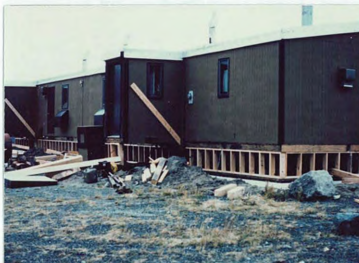
Raising the duplex housing units and furnaces solved the flooding problem. The extra crawl space also makes routine maintenance much easier. (E.V.K. 1984)
