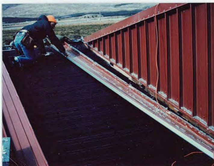
Headquarters roof repair did not completely stop the internal leaking that often results from severe Aleutian storms. (F.Z. 1984)
