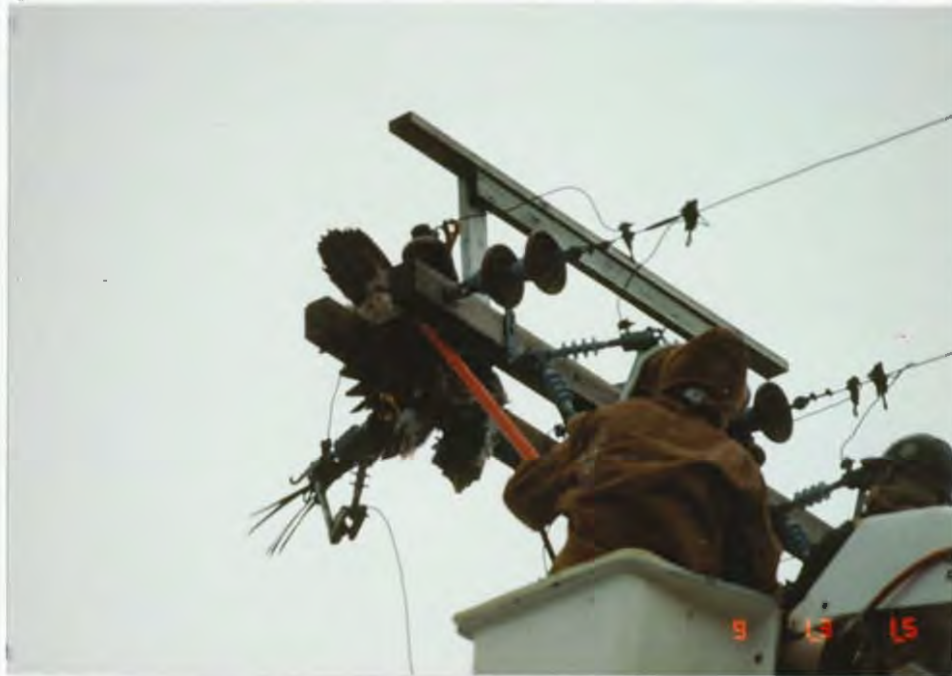
Navy electrical workers retrieve a bald eagle from a pole with an artificial perch. Eagles occasionally get electrocuted on poles with perches but not nearly as often as on poles without perches. JPF.
