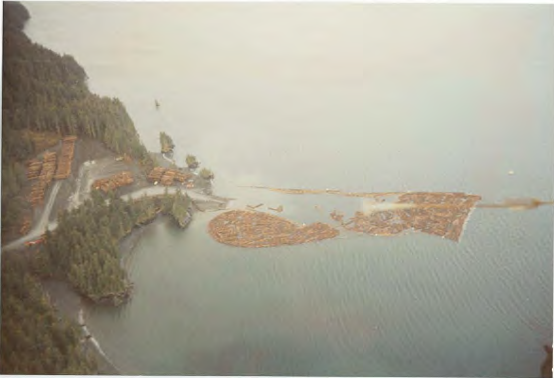
Aerial view of the Koncor operation, Kazakof Bay, Afognak. Nishimoto 1990
