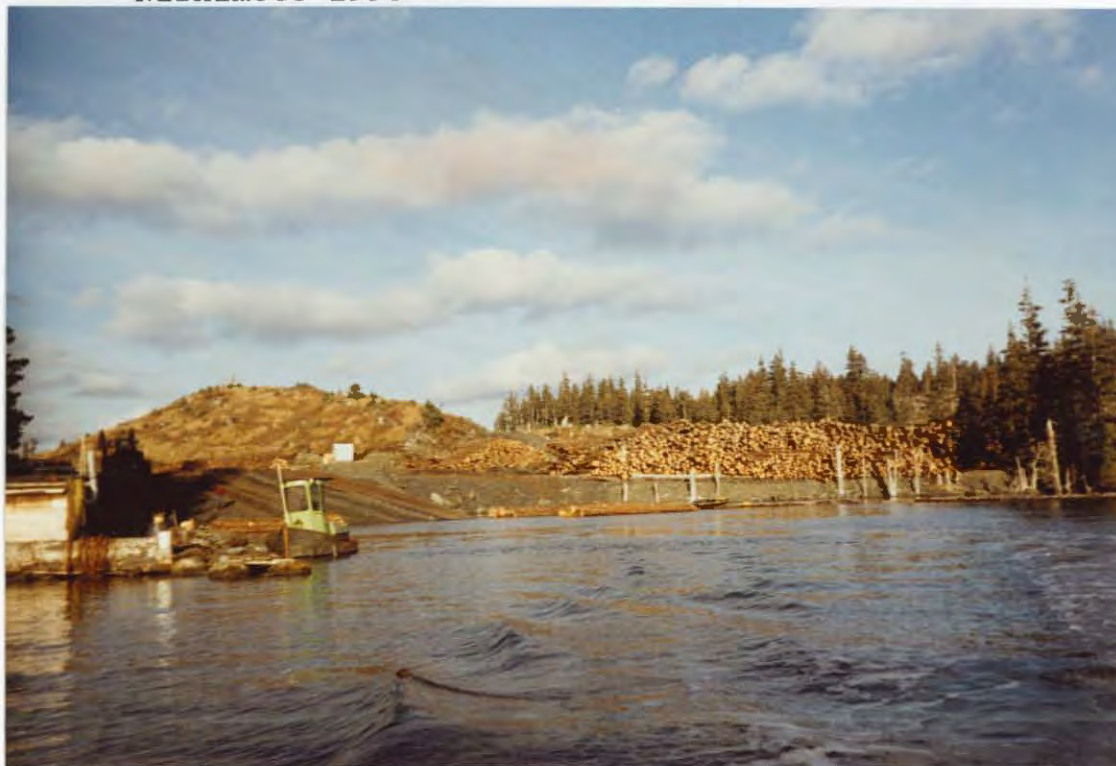
Afognak Native Corporation Log Transfer Facility site, Lookout Cove, Kazakof Bay, Afognak. Nishimoto 1990
