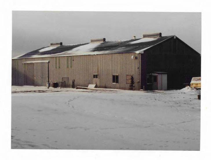
Office space is loacted in this uninsulated, inadequately heated and lighted metal building. Rehab funds are desparately required so staff members are not required to wear parkas and bunny boots to stay warm while working in the offices.
